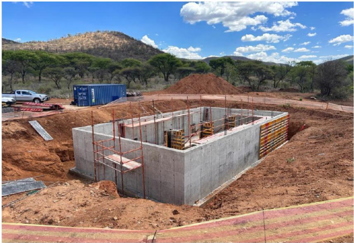
Pump Station 1 Concrete to Walls & Columns
